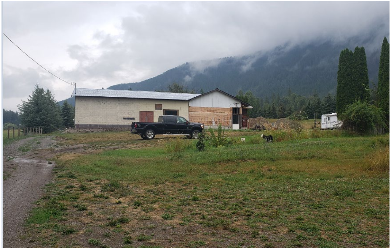
Figure 5: View of the existing farm building and stream from the driveway looking north
